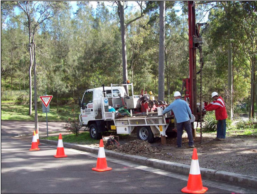
Figure 1: Looking west / north-west towards Bore 1
